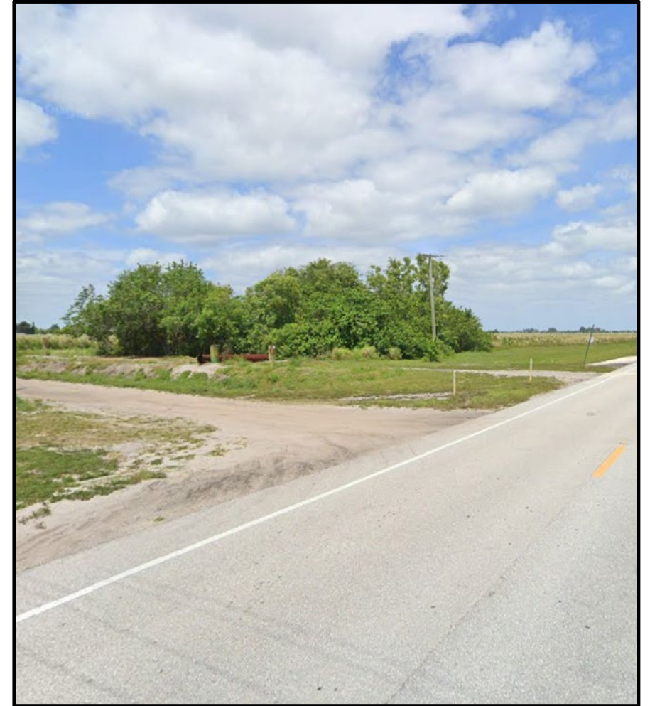
Northbound Lyons Road facing eastbound Smith Sundry Road (pre-construction)
