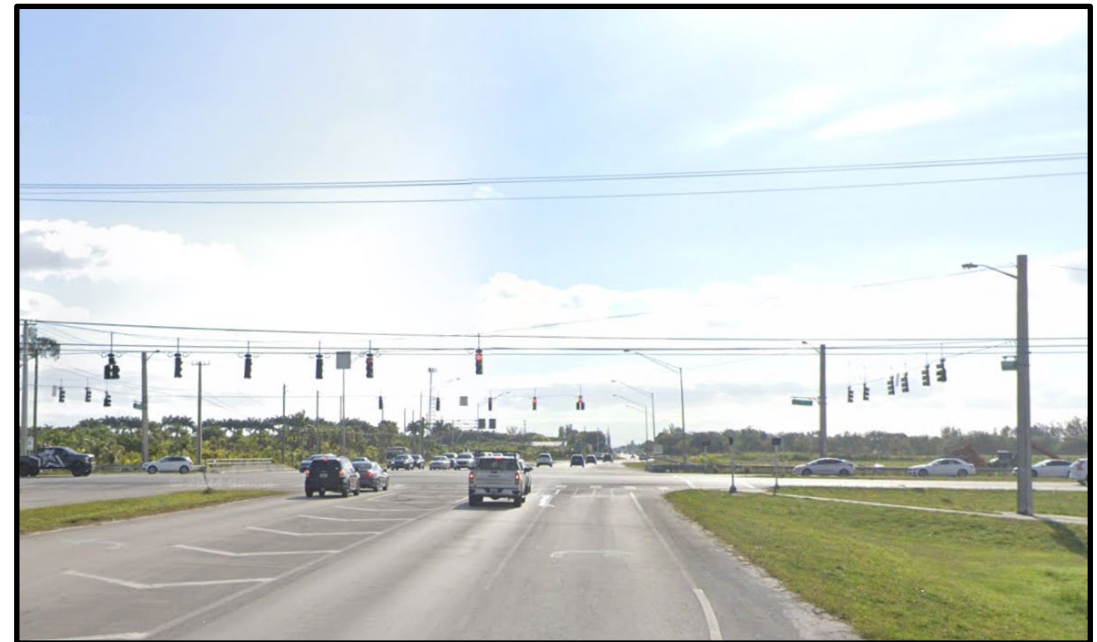
Intersection of SR 806/Atlantic Avenue and SR 7/US 441 facing east (pre-construction)
