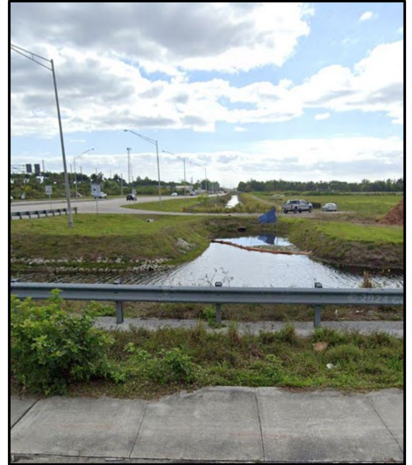
LWDD L-34 Canal facing east (pre-construction)
